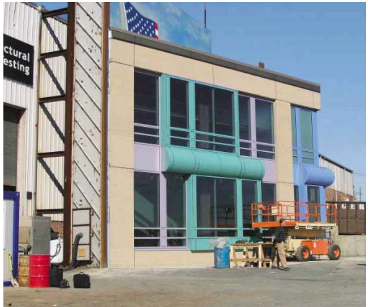
A battery of tests was conducted on a mock-up for the exterior lab wall of the Children's Hospital of Milwaukee, designed by Shepley Bulfinch Richardson and Abbott.
